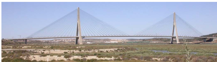
Figure 1. International Guedes de Resende Bridge, Portugal
